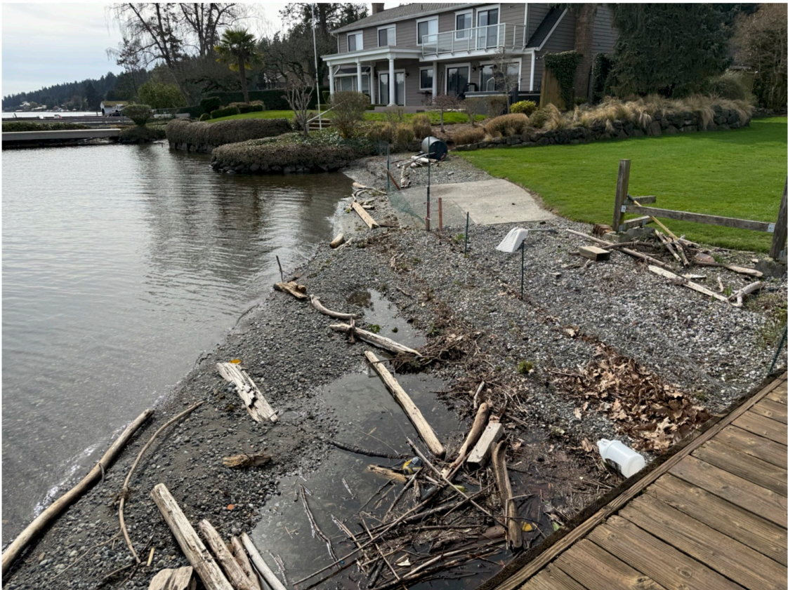
Photo 4 - Existing shoreline south of dock.
