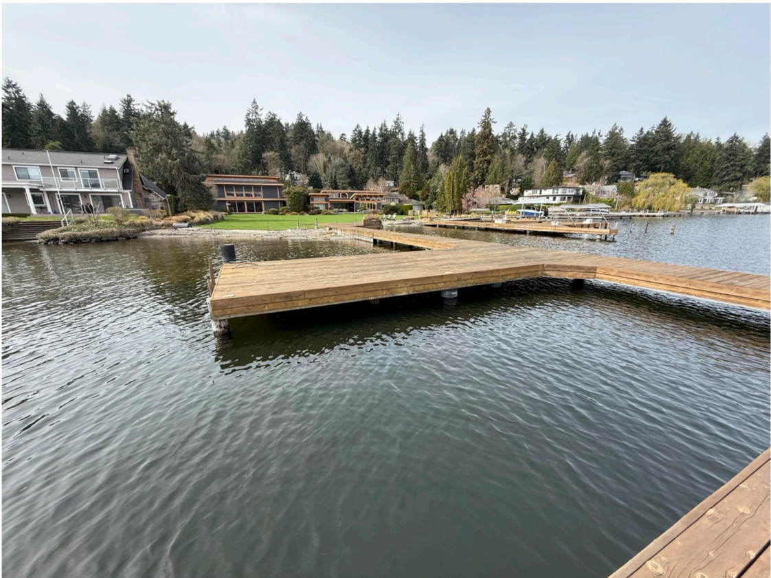
Photo 2 - Existing dock looking landward.
